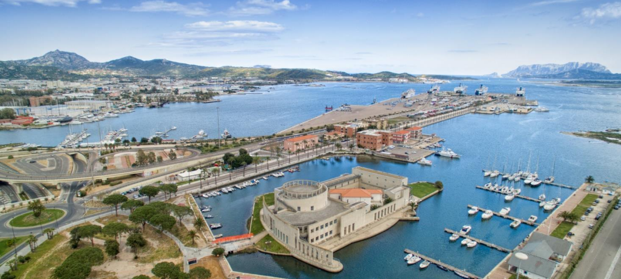
Italian Demo | Olbia Automatic Power Distribution Grid Fault Detection
